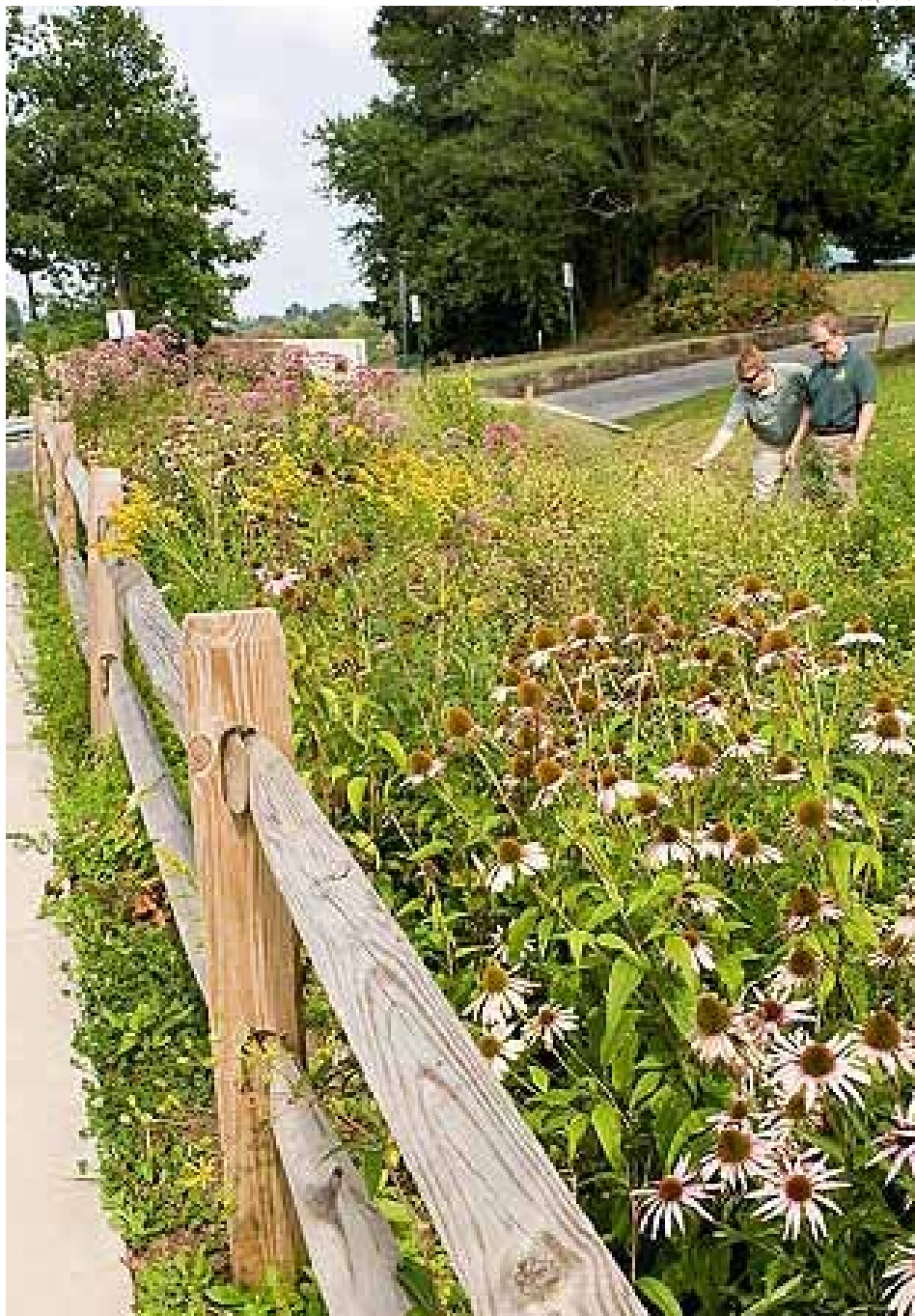
ARS hydrologist Douglas Boyer (right) and Beckley Sanitary Board operations manager Jeremiah Johnson discuss the performance of a rain garden constructed from local materials. The rain garden is being tested for its ability to reduce storm water runoff, increase infiltration, and remove excess nutrients and other pollutants from the runoff water before it gets to streams or other bodies of water.
