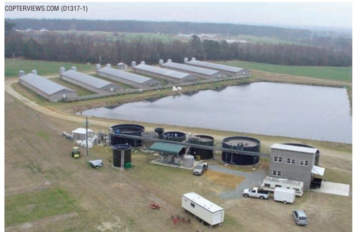
**In Duplin County, North Carolina, this full-scale wastewater-treatment system provided treated swine wastewater for the drip-irrigation study.**
