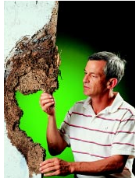
Microbiologist Alan Lax examines carton nest material on insulation and framing damaged by the Formosan subterranean termite.
