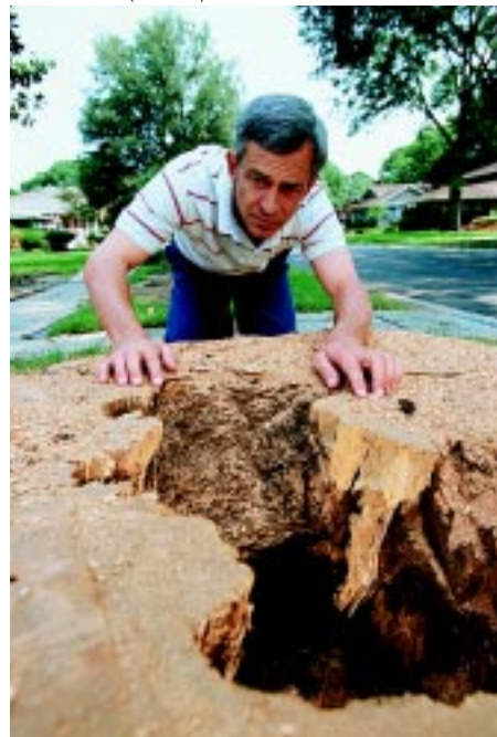
Some remnants of a nest are visible in this cavity, which was hollowed out by Formosan subterranean termites while the tree was still alive. Microbiologist Alan Lax checks the extent of damage.
